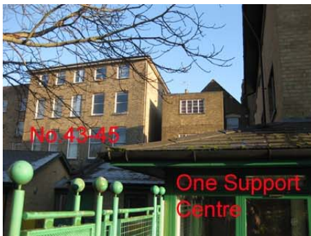
View to rear elevation from One Support Centre
