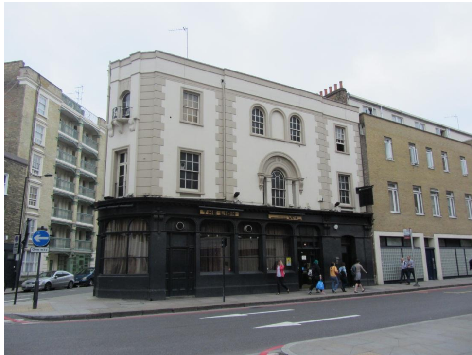
Existing King's Cross Road Elevation
