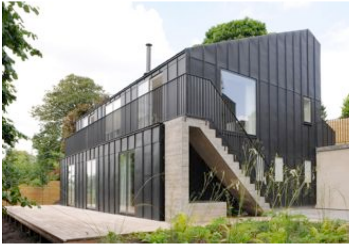
Photograph of zinc cladding
