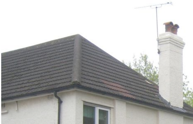
Photo of existing roof
