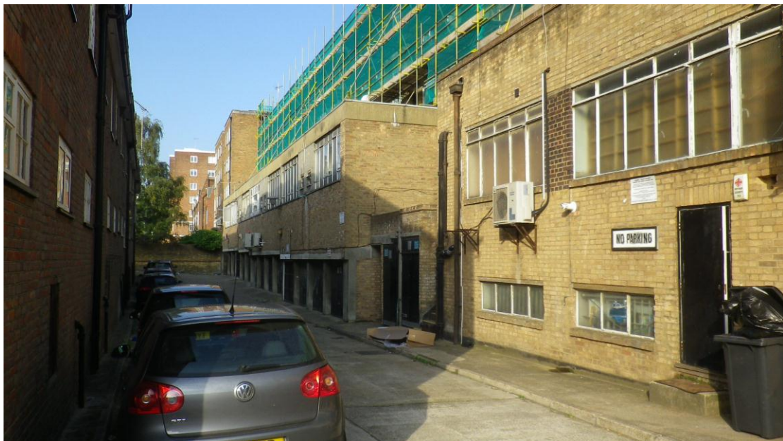
Rear of property from the south (note the existing unit)
