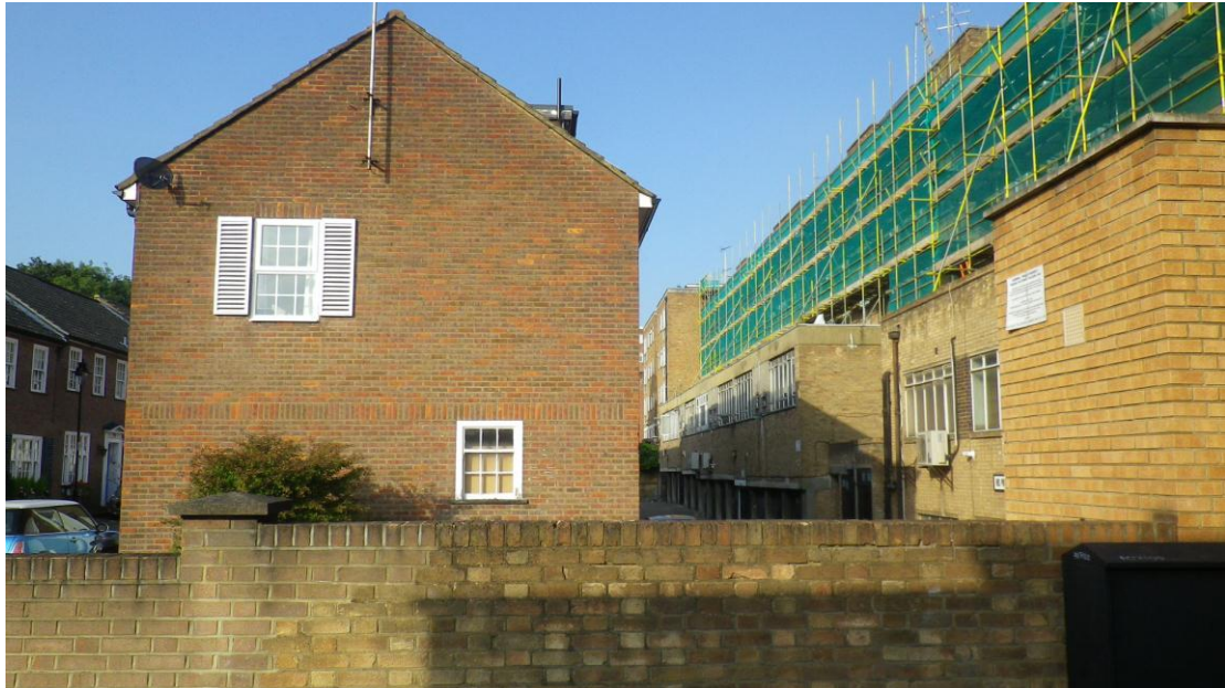
Side of properties on Fairfax Place with rear of Fairfax Road to the right
