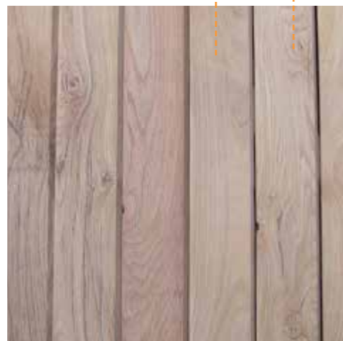
Timber cladding to Entrance door panel and soffit: Vastern Timber Finger jointed Sweet Chestnut cladding
