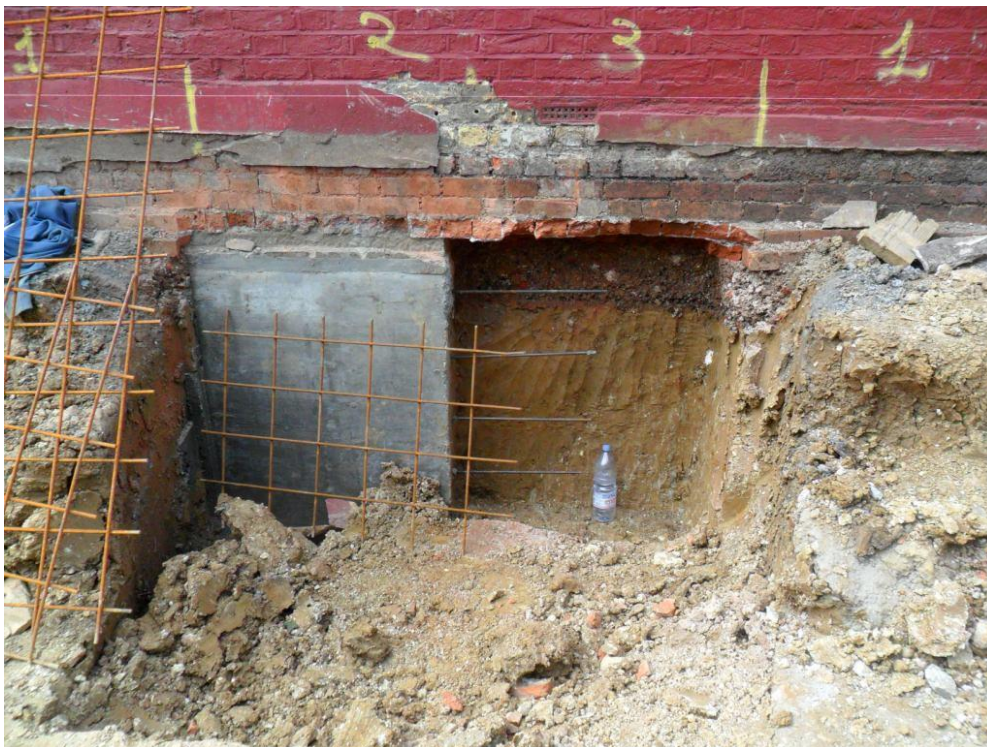
Sequential Underpinning
