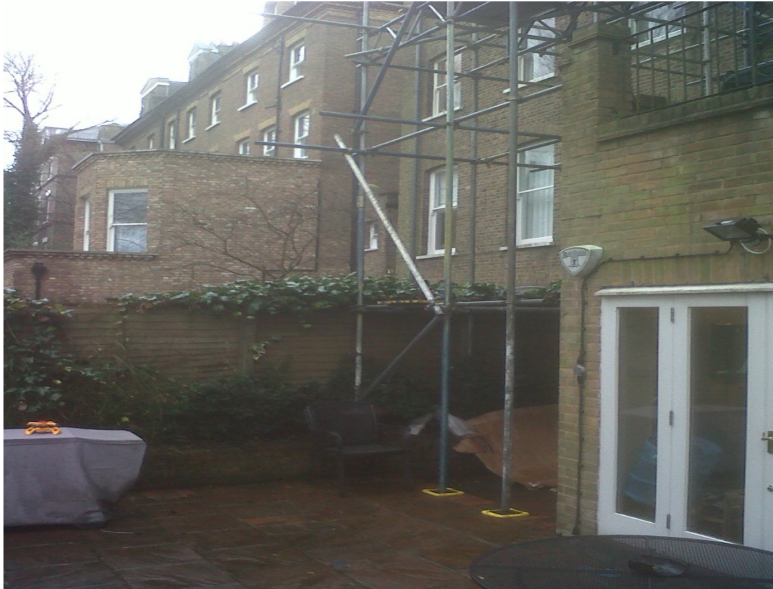
Existing Patio Area
