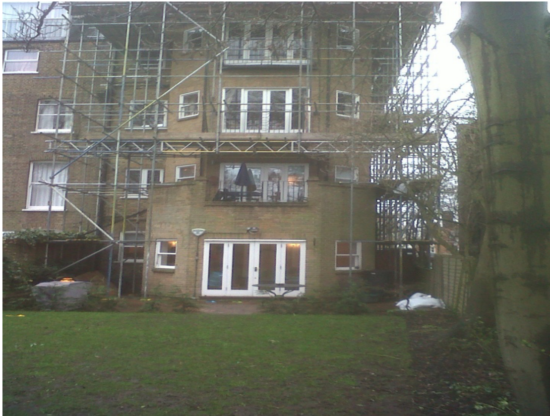
Rear elevation garden space
