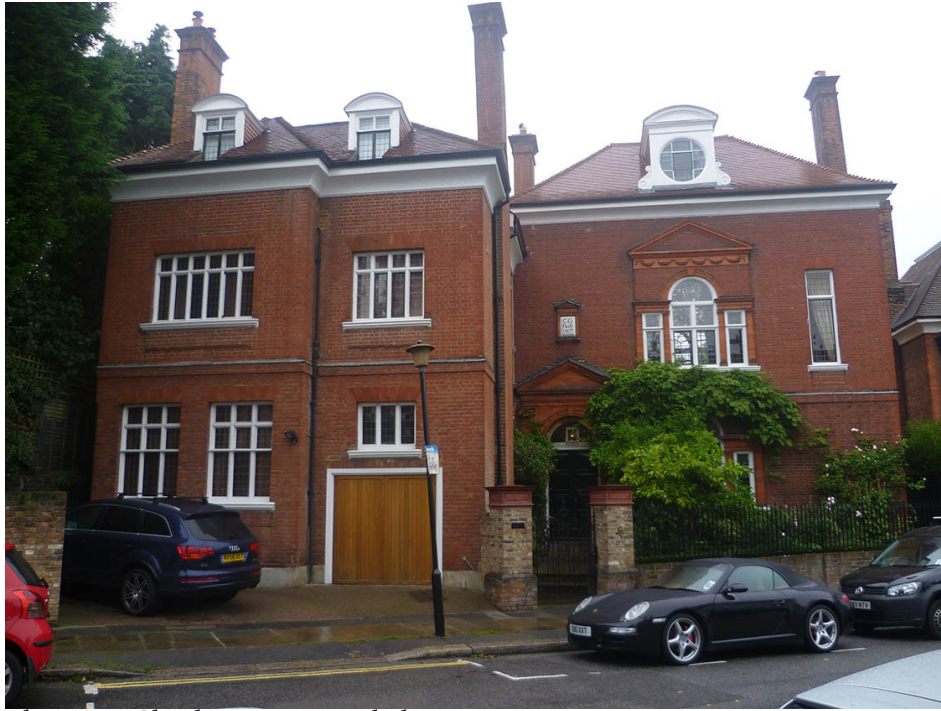
Photo 1 - Charlecote external elevation
