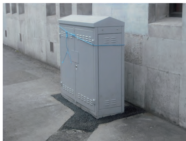
Example of Virgin Media telecommunications cabinet
