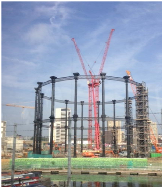
Figures 1 & 2: Gas Holder No.8 re-erection on Development Plot N2
