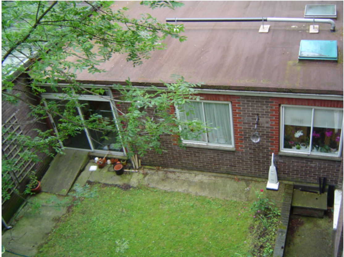
Rear extension at no 11
