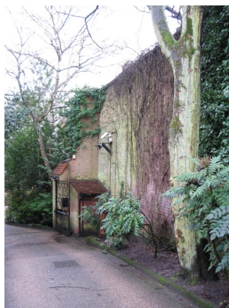
4-5m high wall along the site's southern boundary
