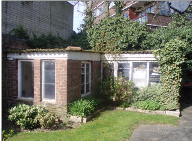
Buildings located in the rear gardens
