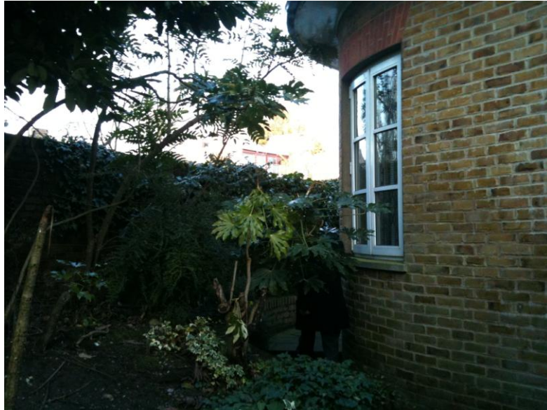
First floor extension
