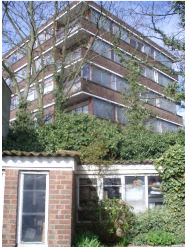
Block of flats to the rear of the application site.
