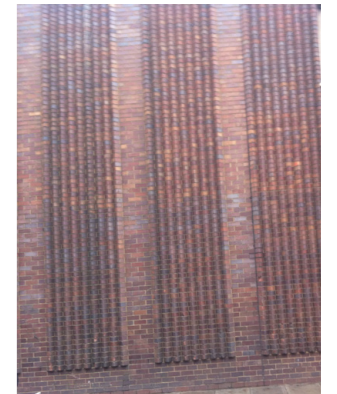
Panels of dog-tooth brickwork
