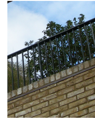
Metal railings on brick walls
