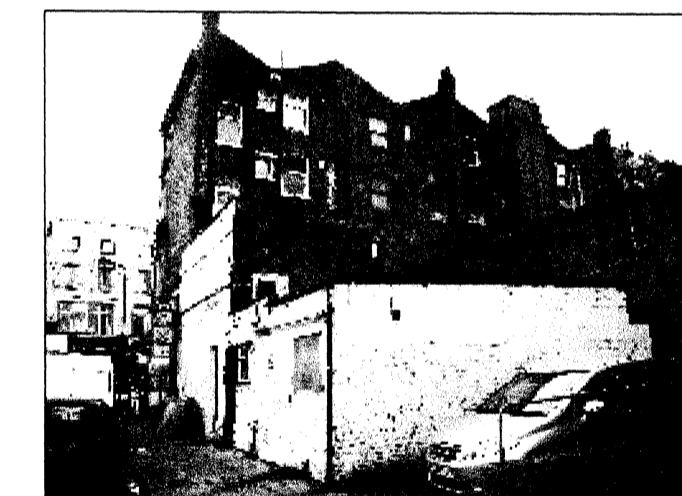
PHOTOGRAPH: REAR ELEVATION
