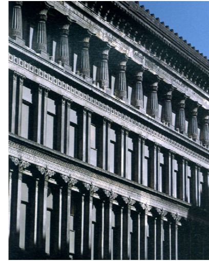
The Egyptian Halls, 84-100 Union Street, Glasgow, Scotland Alexander 'Greek' Thomson, (1817-1875) 1870-72, (new commercial premises with shops below)
