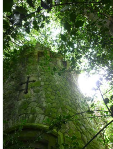
P8 Milner folly on north side with missing stone work round the turret
