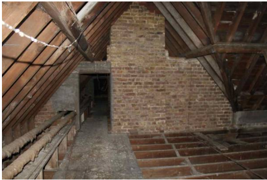
P5 Large roof void
