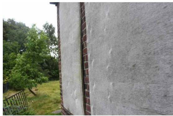
P4 Boarded-up window on northern elevation
