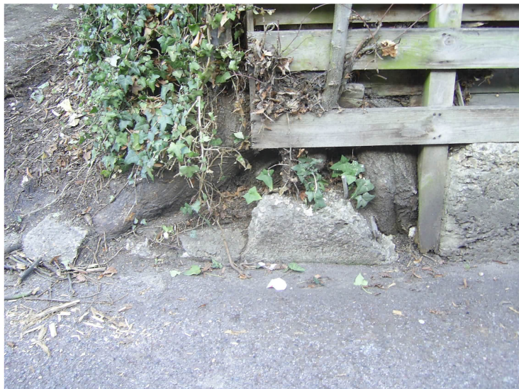
Part of the rooting system of T1 is visible at the present entrance to the site.
