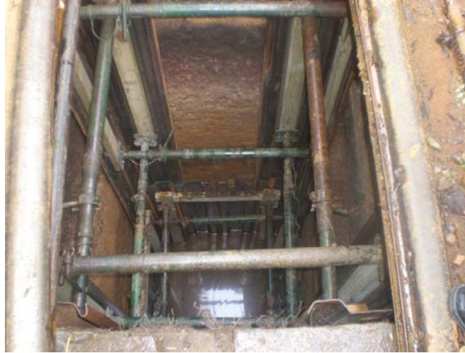
Figure 15 Propping
