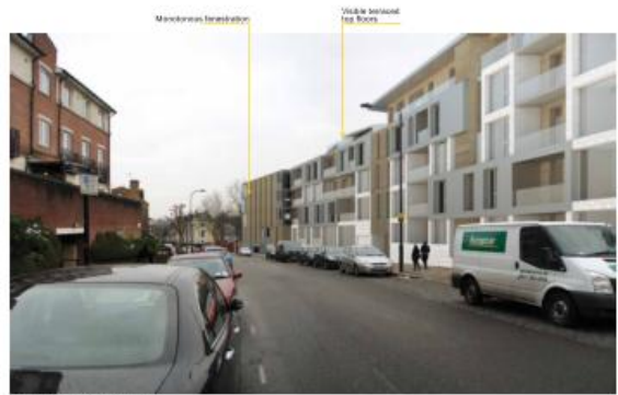
View along Iverson Rd, looking west pre-application scheme_march 2013
