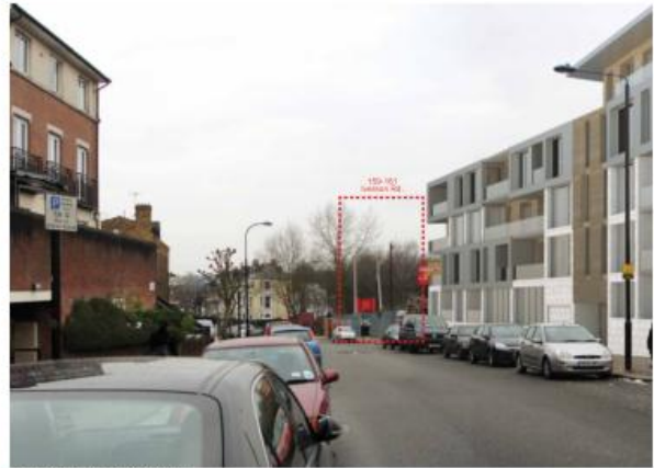
Existing view along Iverson Rd, looking west with consented scheme for 163, Iverson Road
