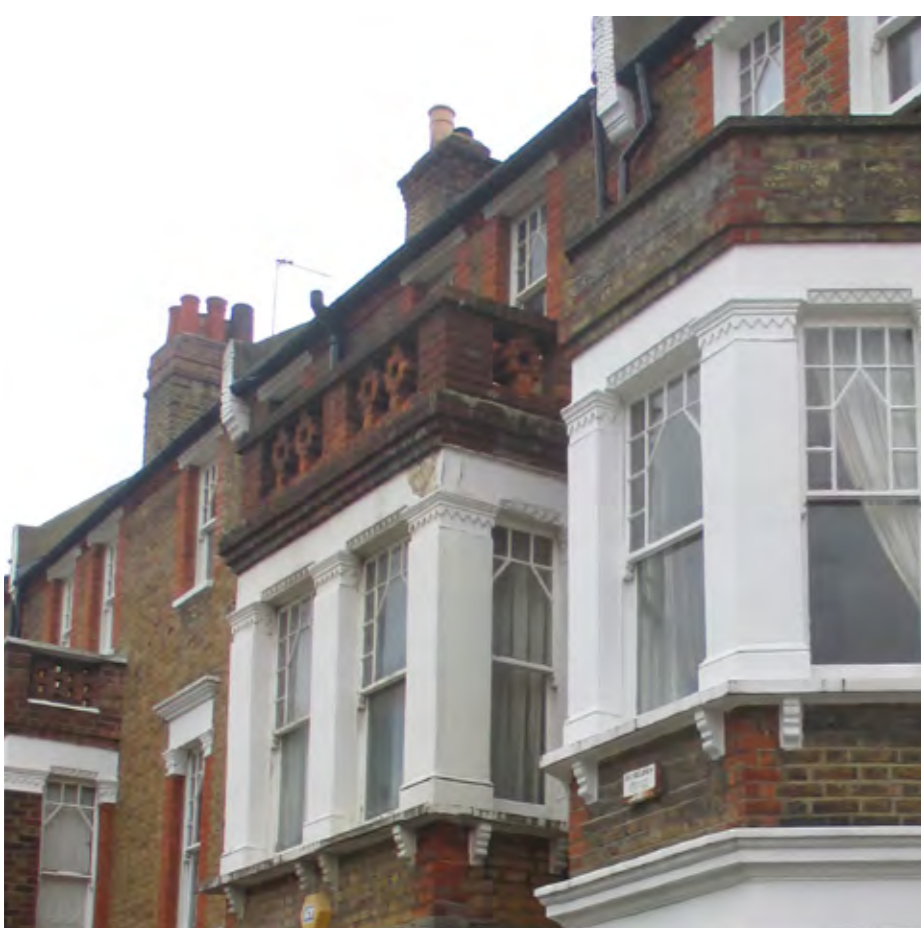
Parapet bays with top storey opening out over
