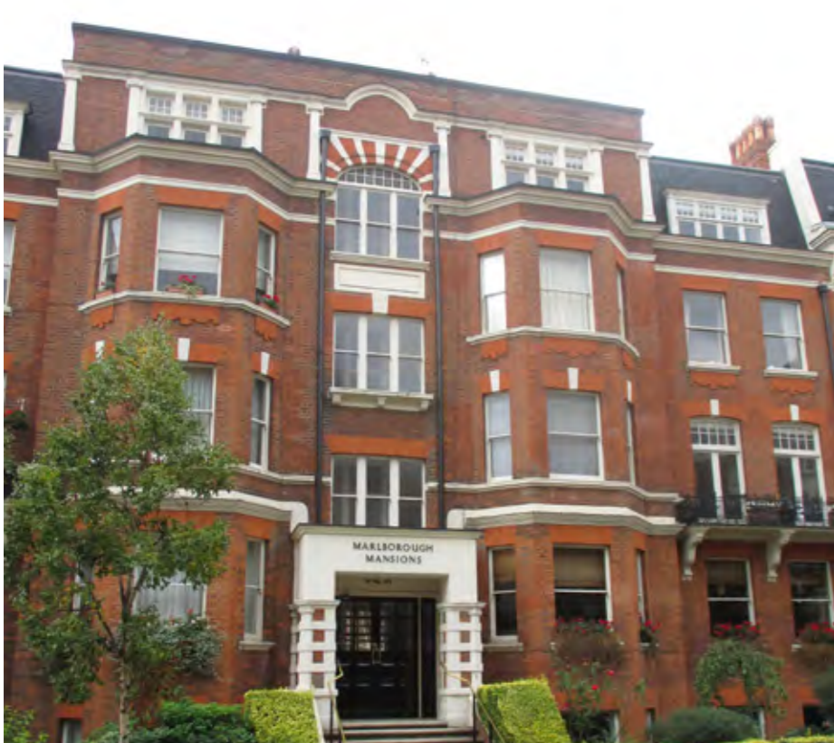
Flat roof behind bays creating sense of grandeur
