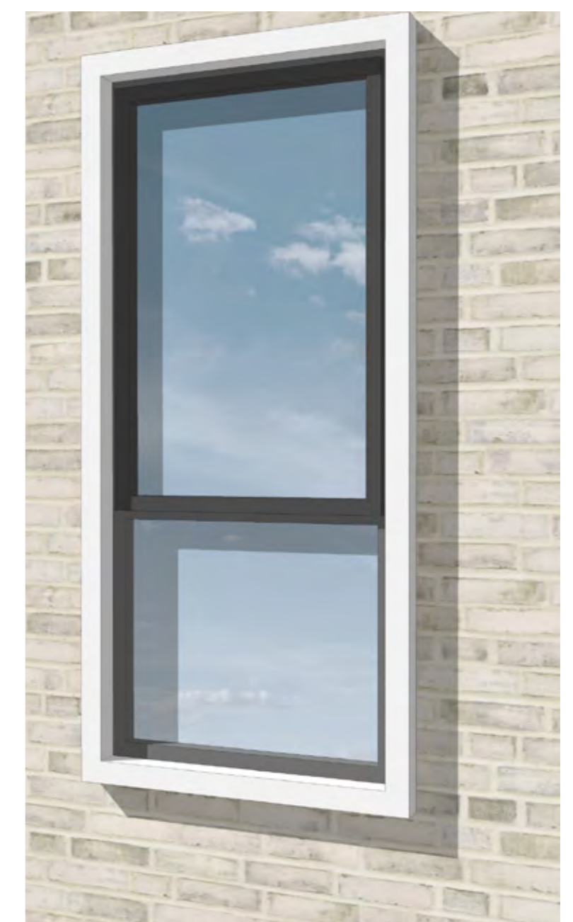
The darker aluminium opening light creates added detail. The size and depth of the reveal can be seen to draw parallels to the pronounced cills on the neighbouring mansion blocks
