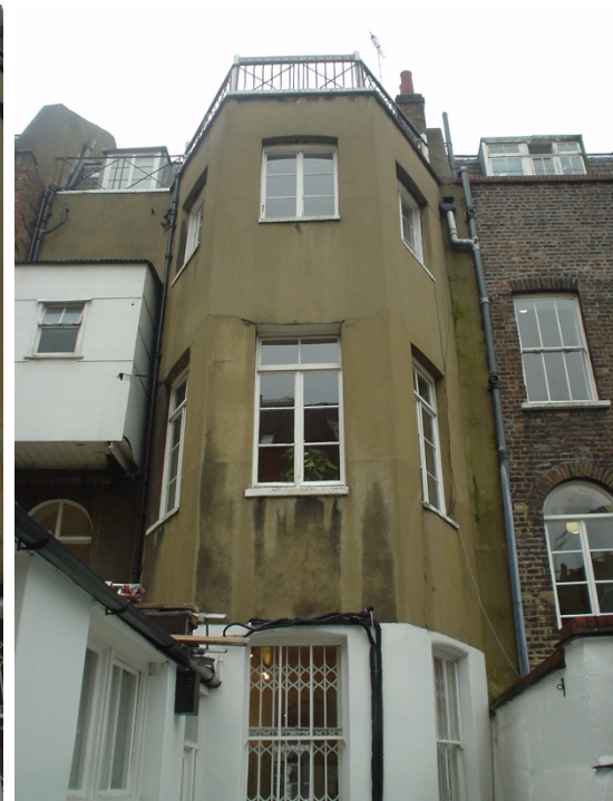
Photo 4: Rear view of number 31 and 32 Percy Street.
