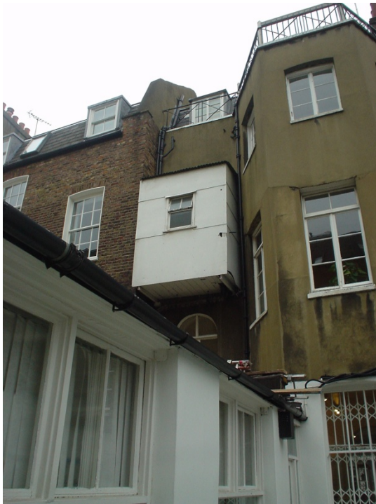
Photo 3: South easterly view of the adjoining buildings of 30 and 31 Percy Street.
