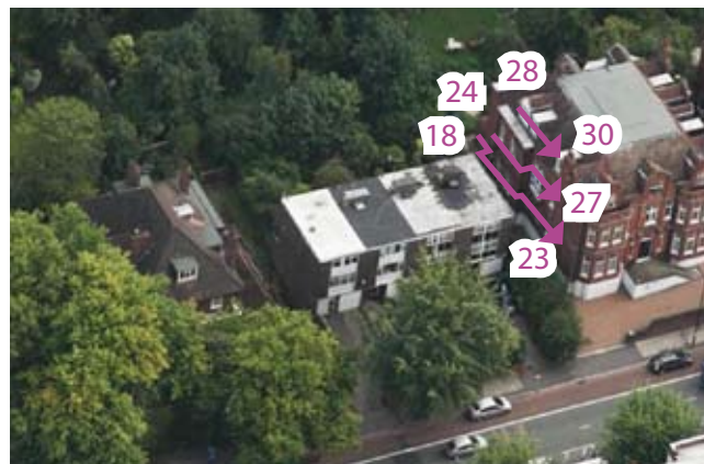
Potentially affected windows on 262 Finchley Road
