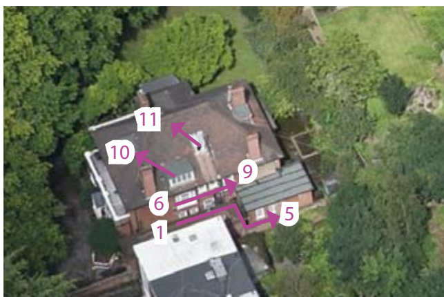
Potentially affected windows on 38 Heath Drive
