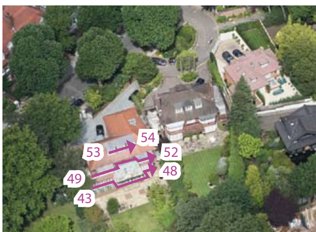
Potentially affected windows on 37 Heath Drive
