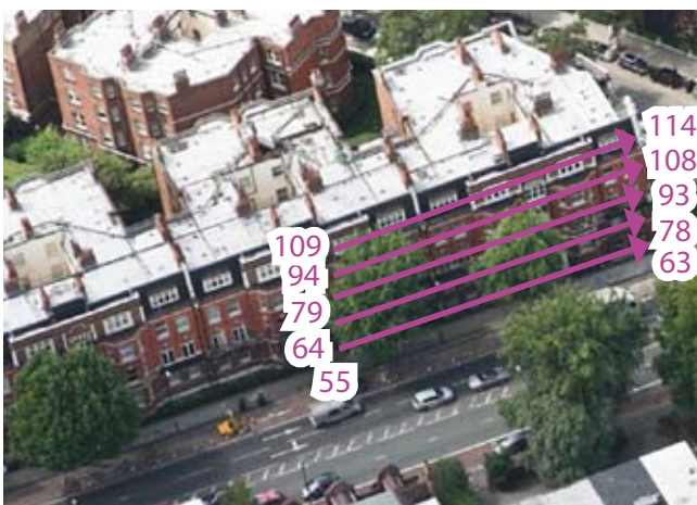
Potentially affected windows on residential building to the south
