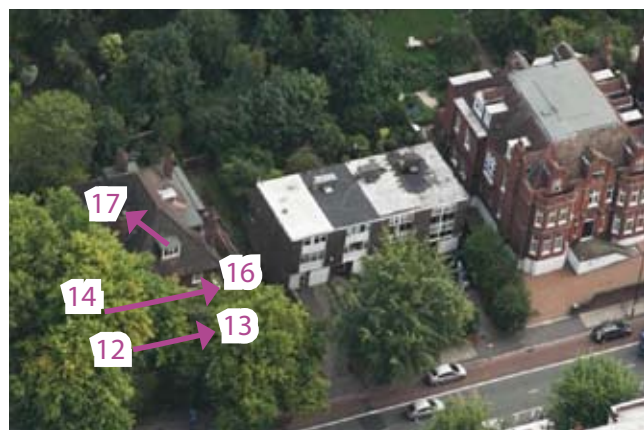
Potentially affected windows on 38 Heath Drive
