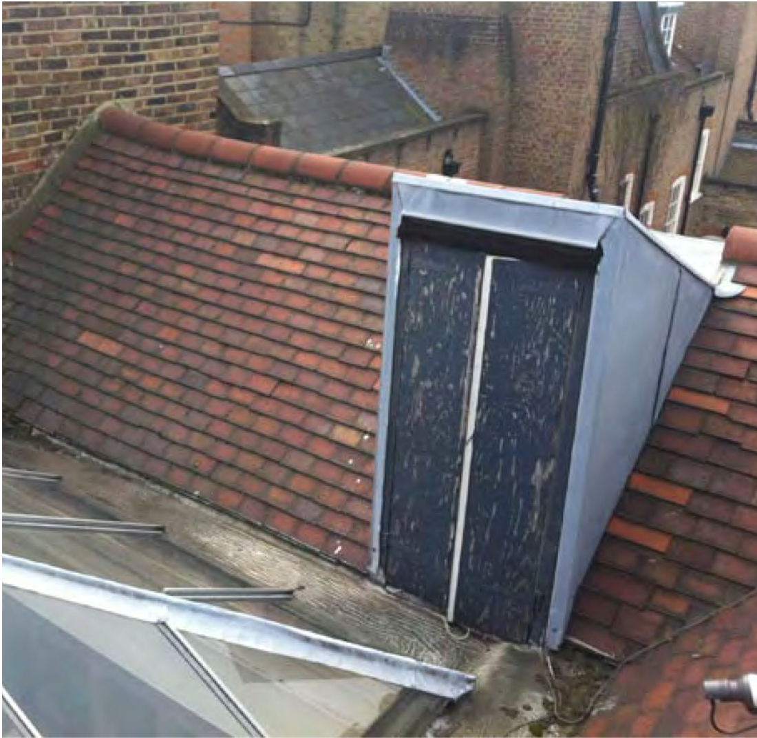
Existing roof access
