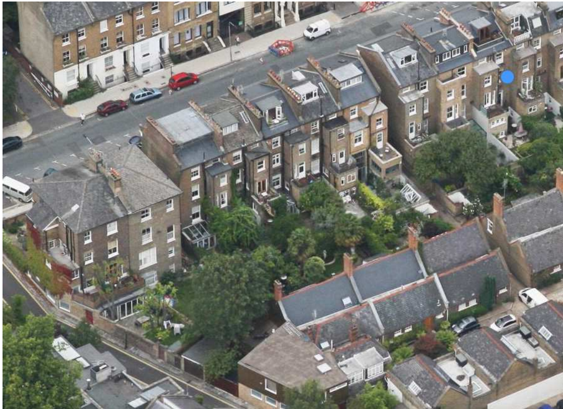
Aerial view. Primrose Hill Studios at the bottom of the image. The application site is the second terrace property on the left hand side.
