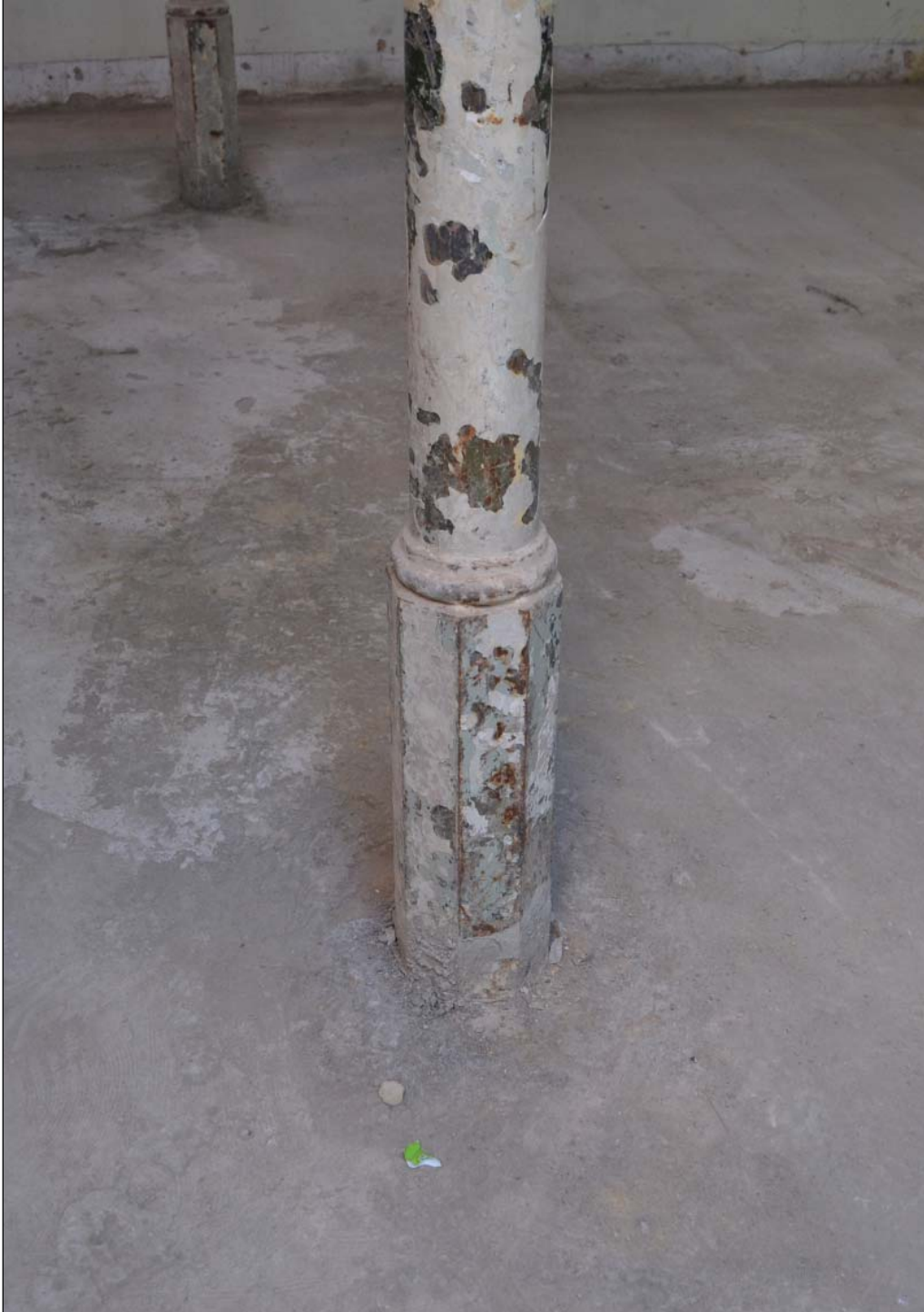
13. Slender cast iron column base
