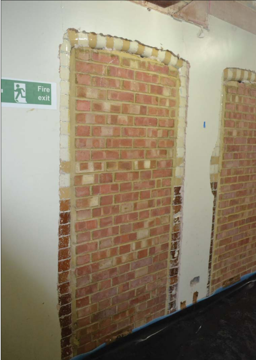
14. Glazed brick arch infilled
