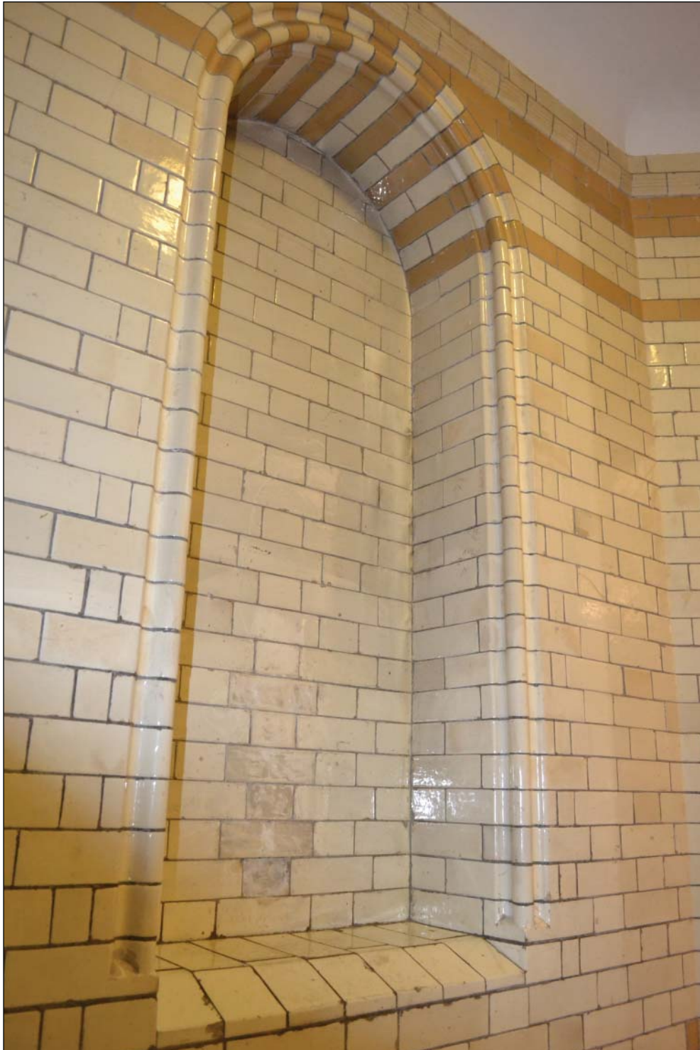
3. Niche within stair compartment
