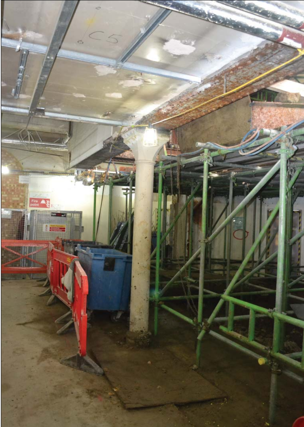
11. 0124 large cast iron column
