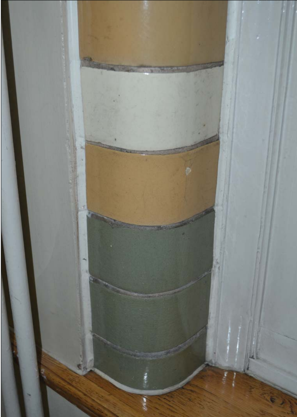
1. Ground floor, showing glazed bricks in beige, cream and green
