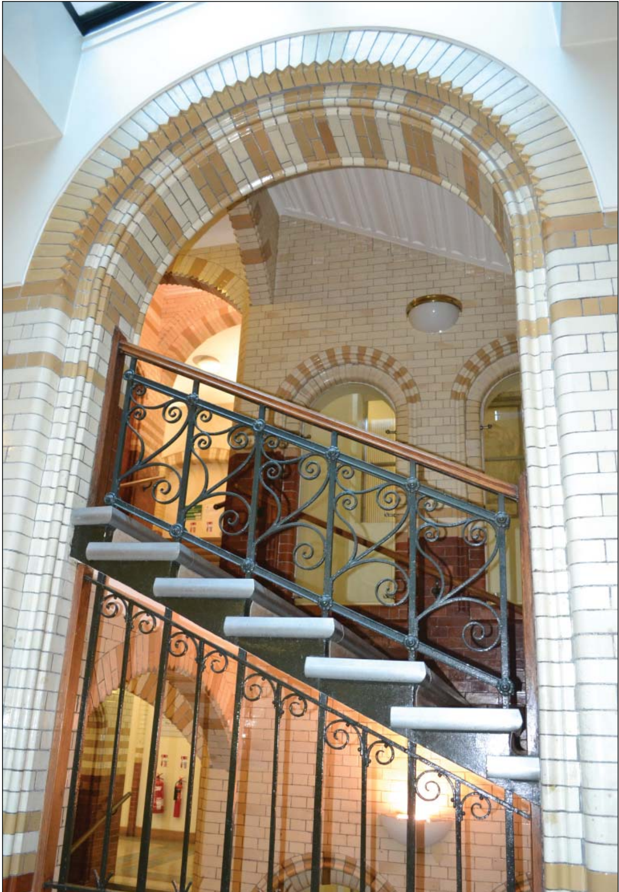
7. Arch through to stairs, ground floor
