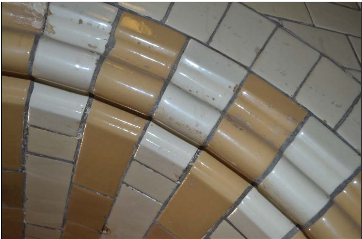
4. Decorative roll mouldings typical of detailing within stair compartment
