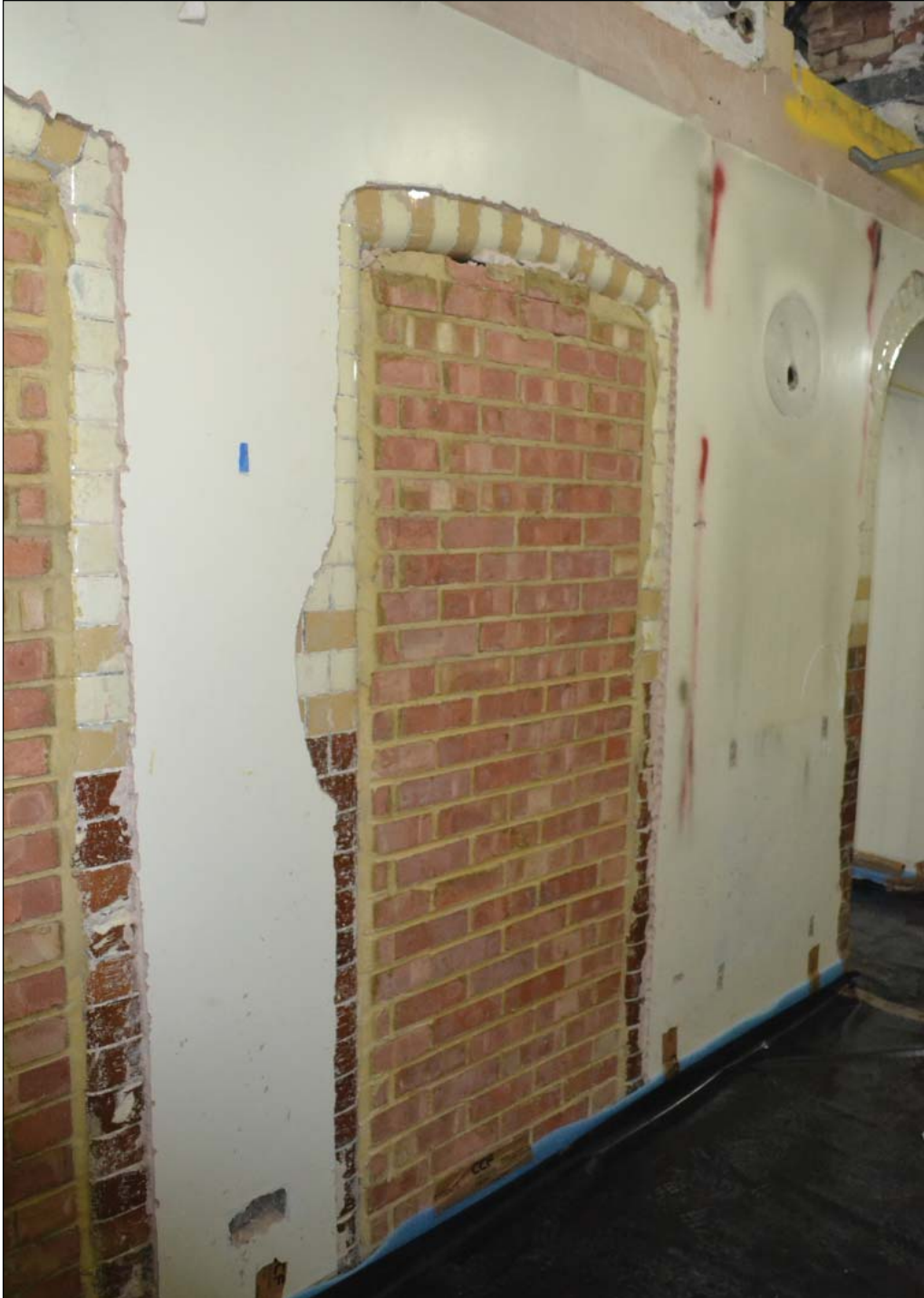
15. Glazed brick arch infilled
