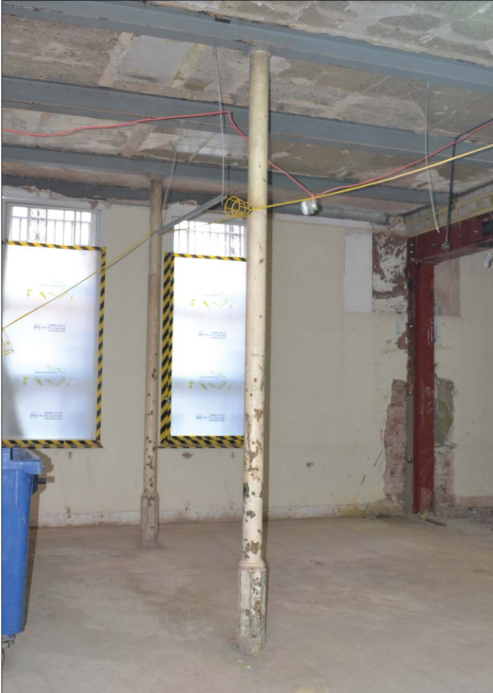
12. Slender cast iron column
