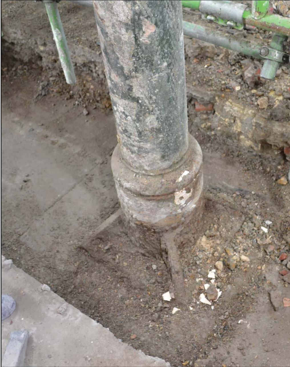
10. Large cast iron column base
