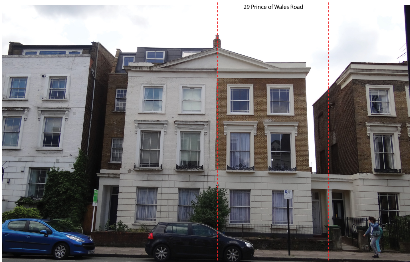
FIG 3.2 Frontage of the site and adjacent properties.
