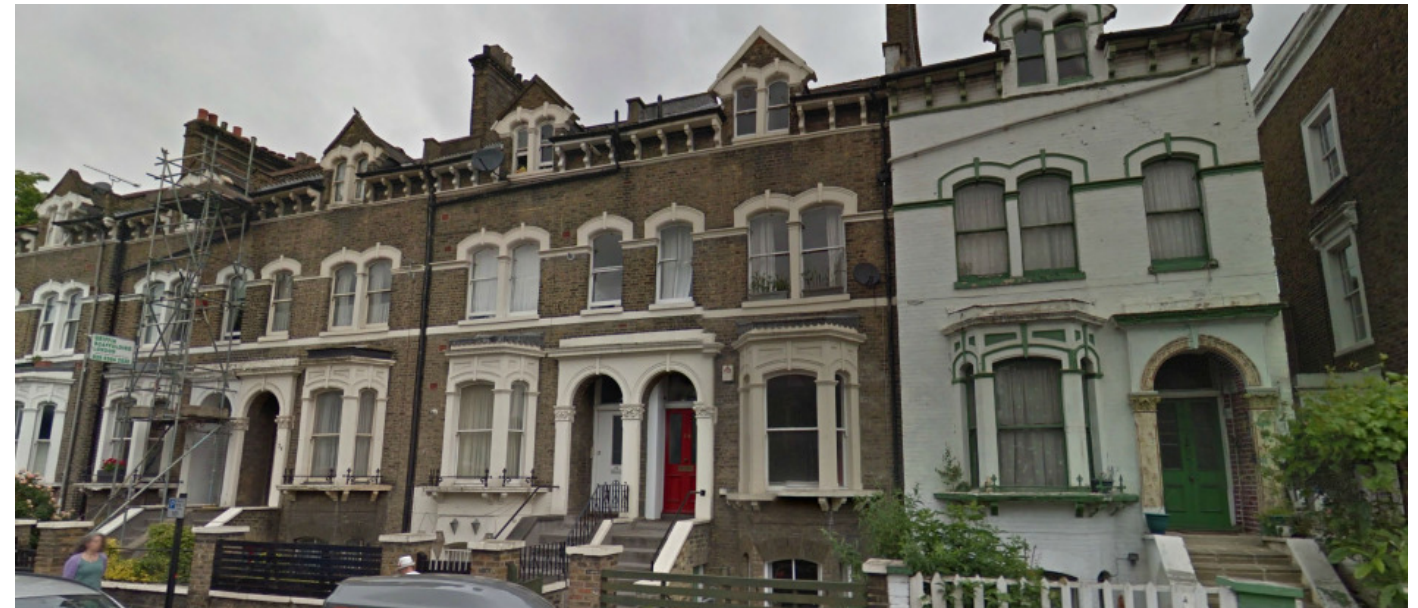
FIG 5.2 View from door of 29 Prince Of Wales Road
