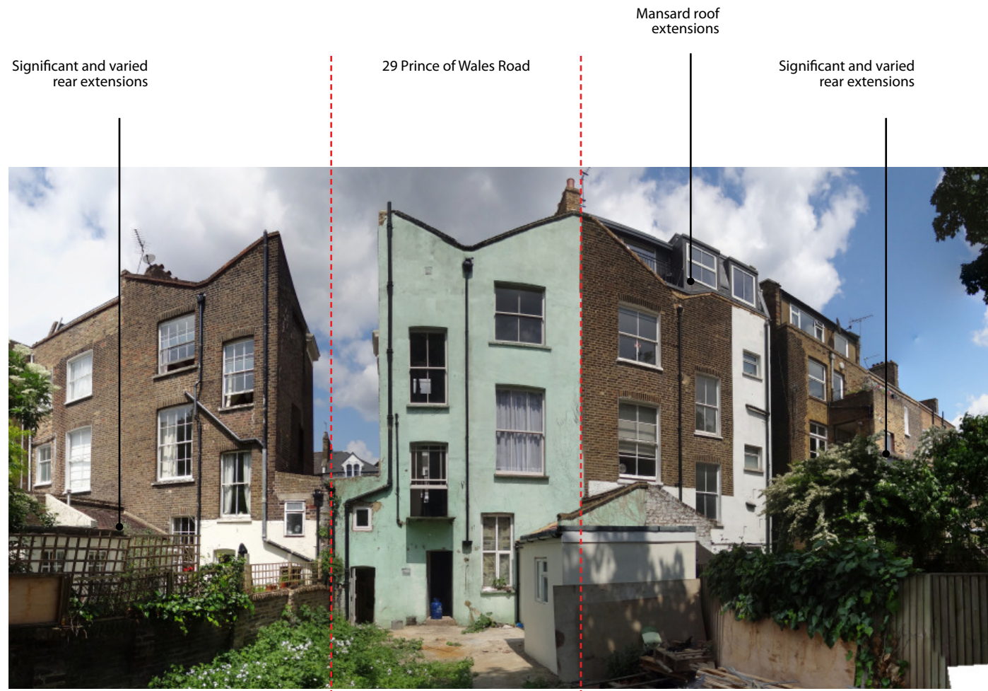
FIG 4.1 Rear Elevation of 29 Prince of Wales Road
