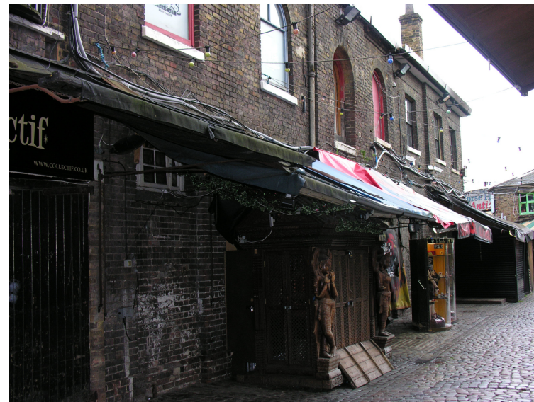
Figure 2: Tack Room east elevation showing widened opening on LHS and replaced windows on the first floor.
