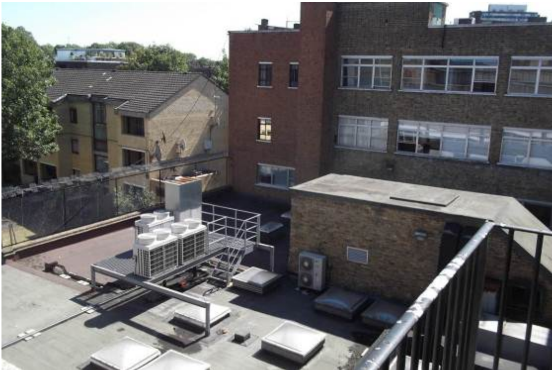
Plate 4. Roof of building to east, with four storey building section beyond.
