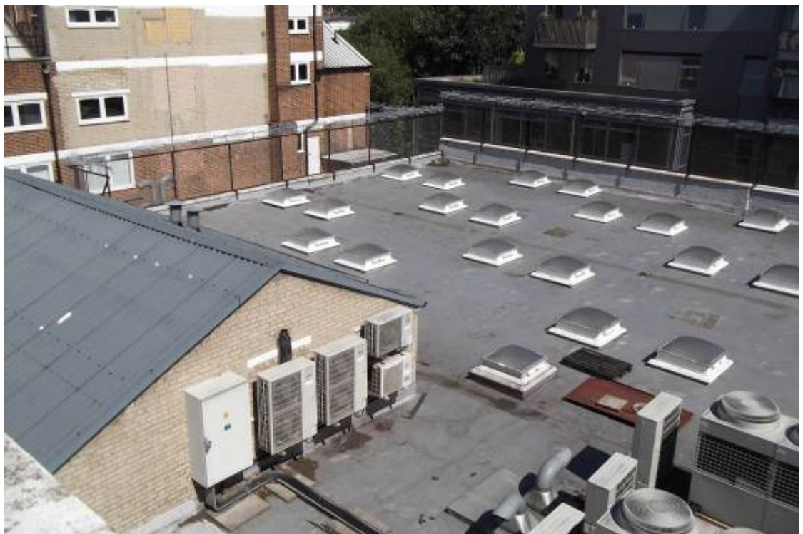
Plate 3. Roof top with skylights and service building to north.
