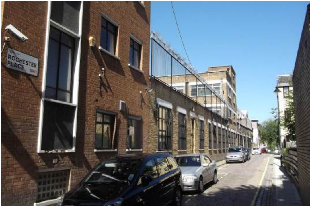
Plate 1. Exterior of the building to the north along Rochester Place.
