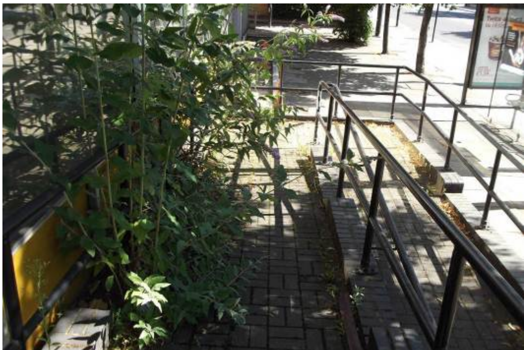
Plate 6. Ephemeral vegetation on ramp leading from Camden road to the entrance to the building.
