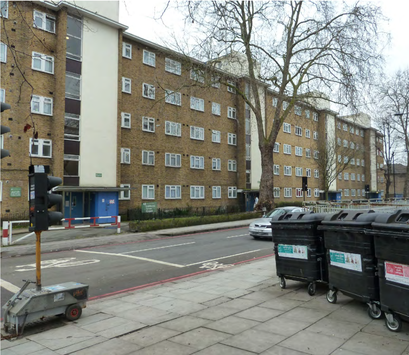
Appendix 2.19: The St Pancras Way elevation of Bernard Shaw Court.
