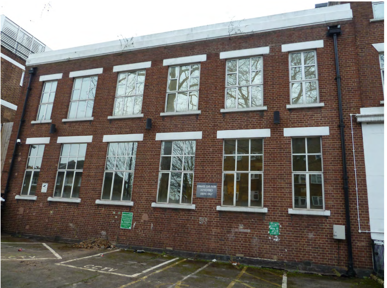
Appendix 2.10: Frontal view of the western part of the frontage.
