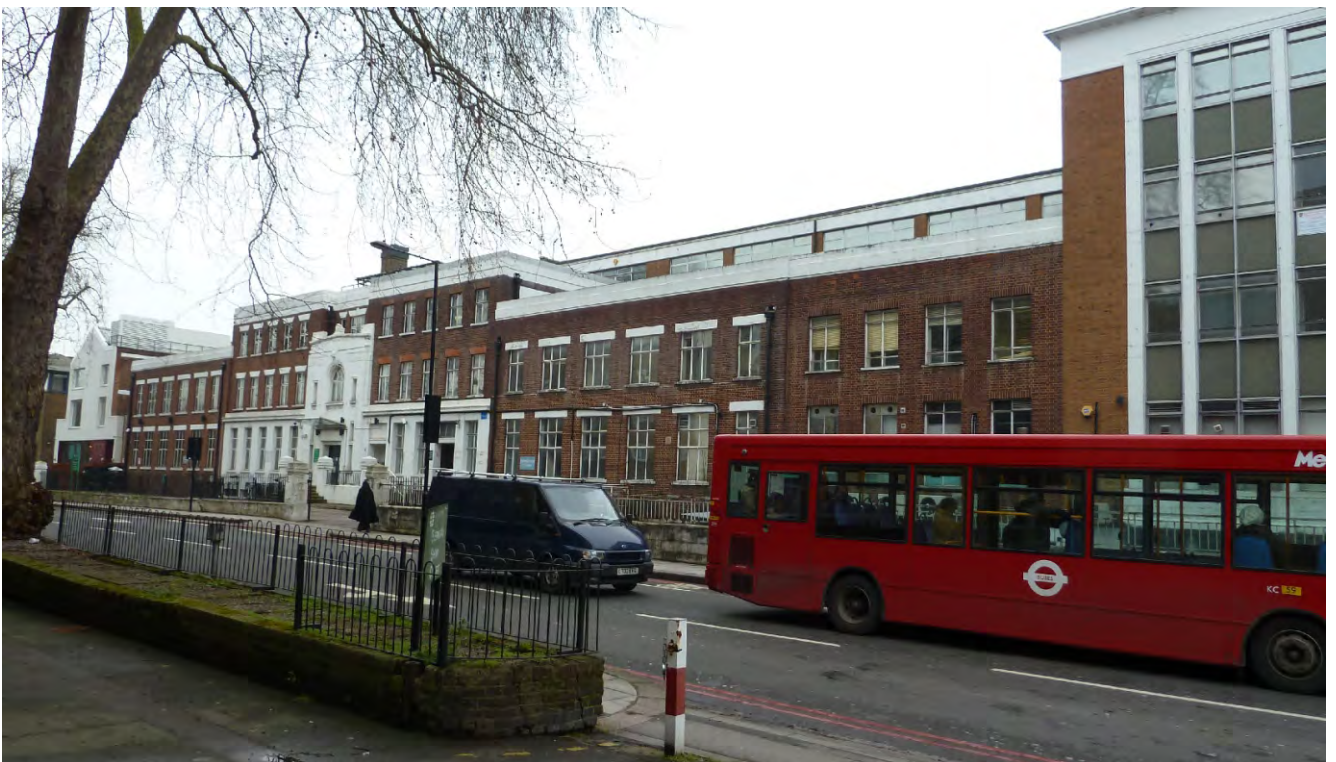
Appendix 2.6: The St Pancras Way frontage of the application site, viewed from the east, outside of the Camden Broadway Conservation Area.
