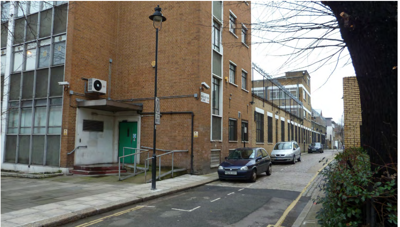
Appendix 2.17: General view northwest along Rochester Place from Camden Road.
