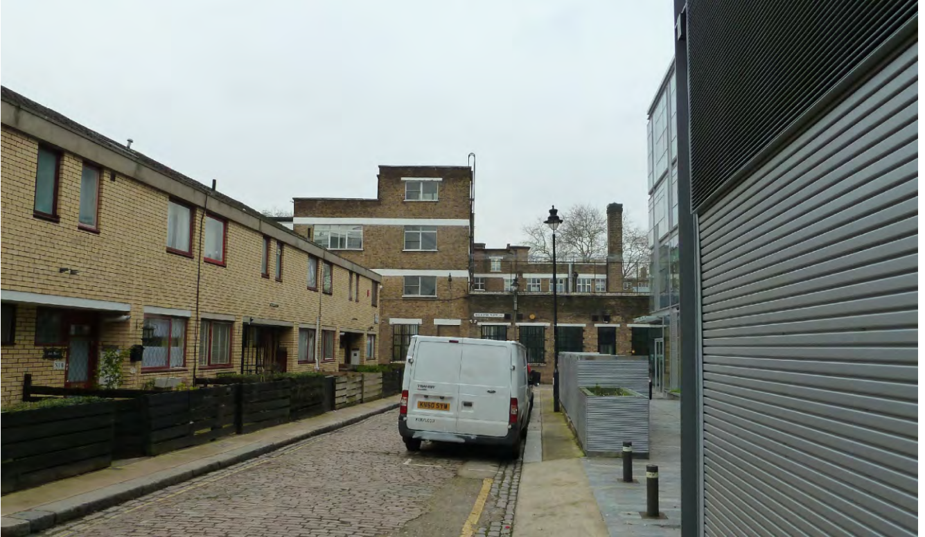
Appendix 2.15: General view southwest towards the application site, along Rochester Mews.
