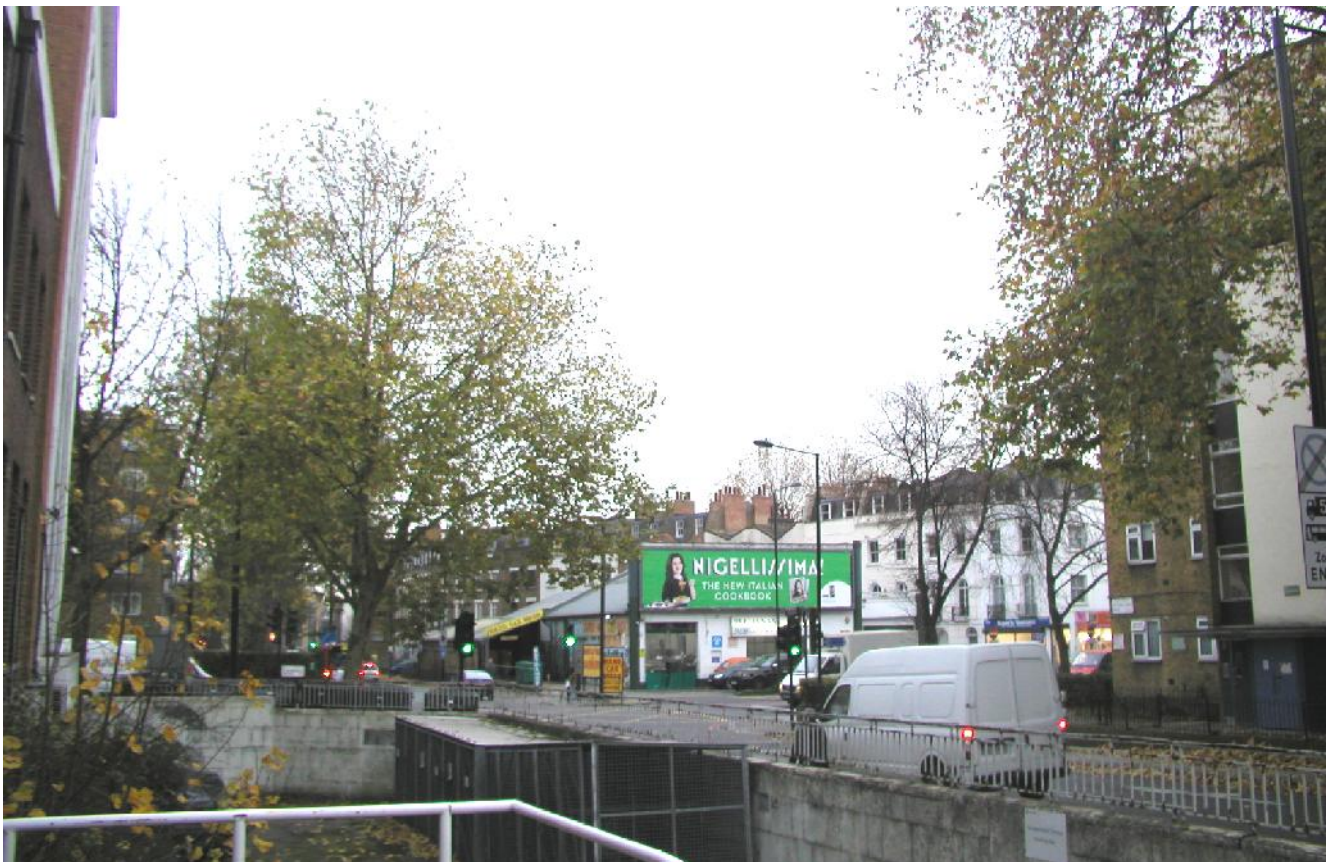
P4: View south east showing ramp down to basement 5m from plane T9.
