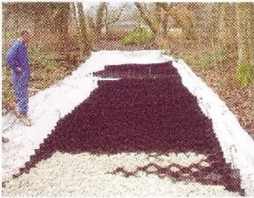
CellWeb during installation.
