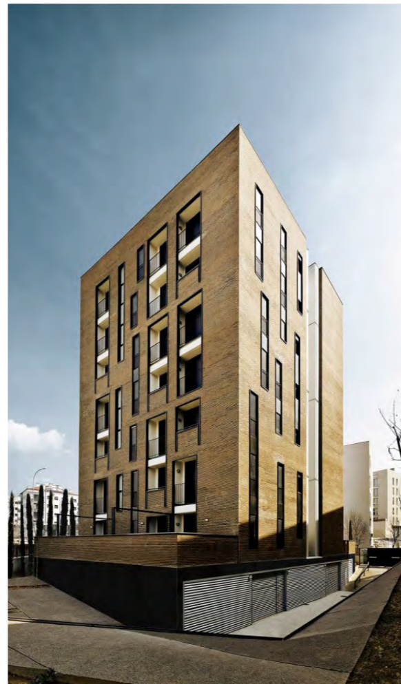
brickwork + opening proportions
