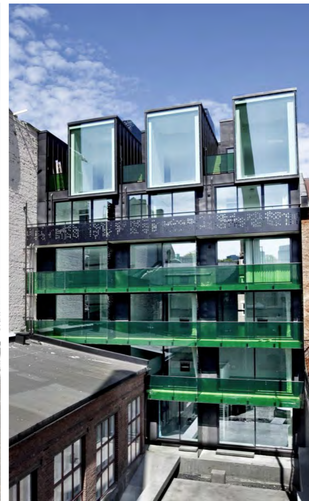
roof level penthouses
