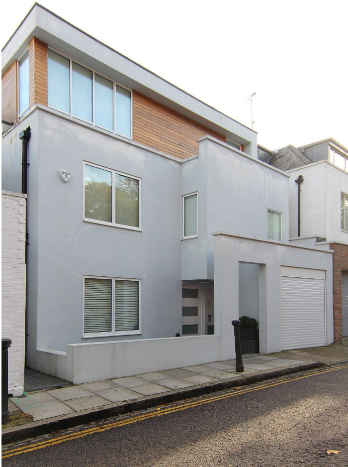
EXISTING FRONT VIEW
