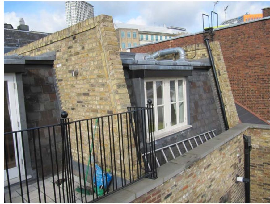
02 - Existing mansard roof construction with dormer windows
