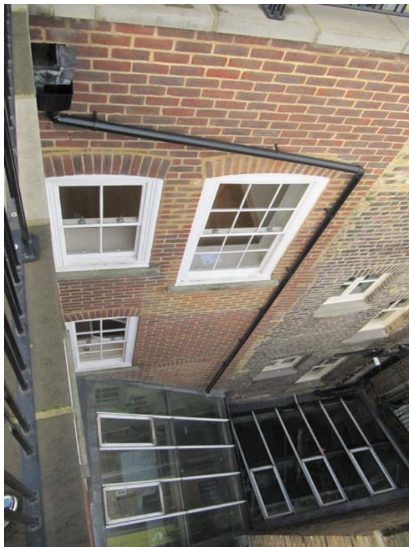
04 - Existing view from terrace to roofs below
