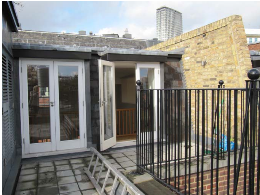
01 - Existing roof terrace with terrace doors
