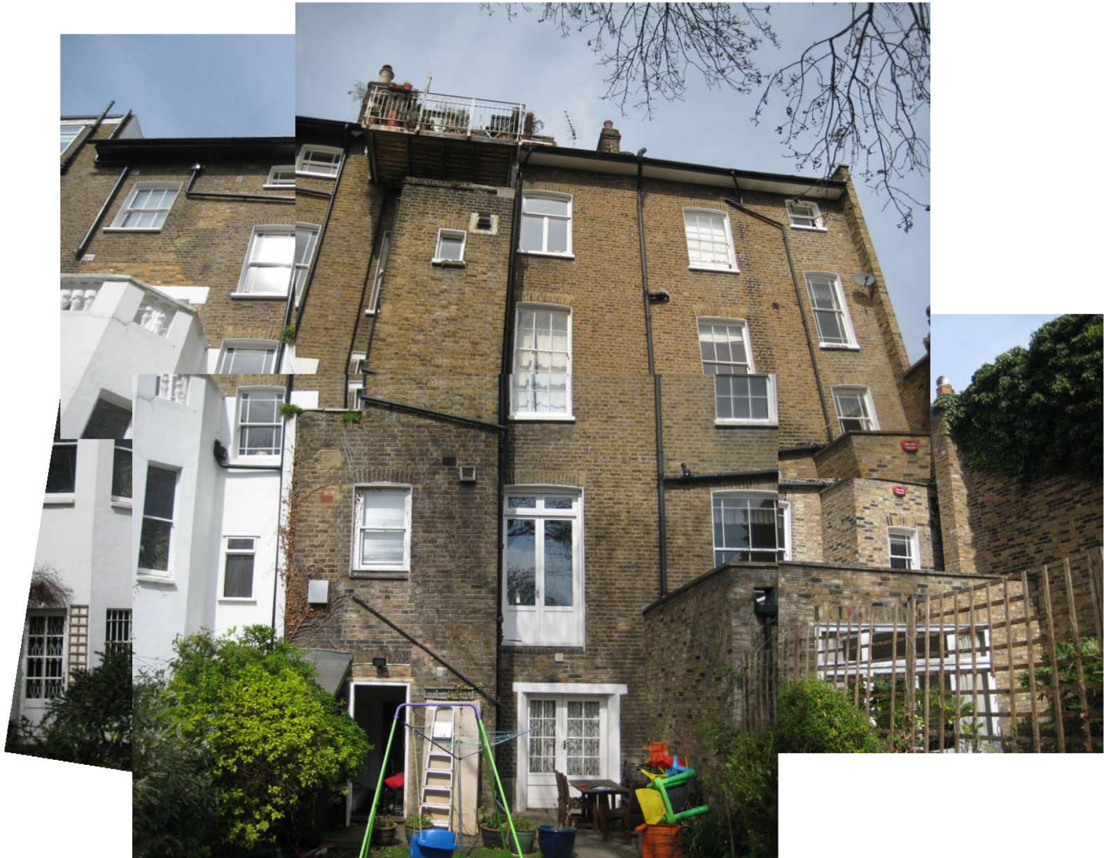
View of the rear of Nos. 20, 21 and 22 Steeles Road London NW3
