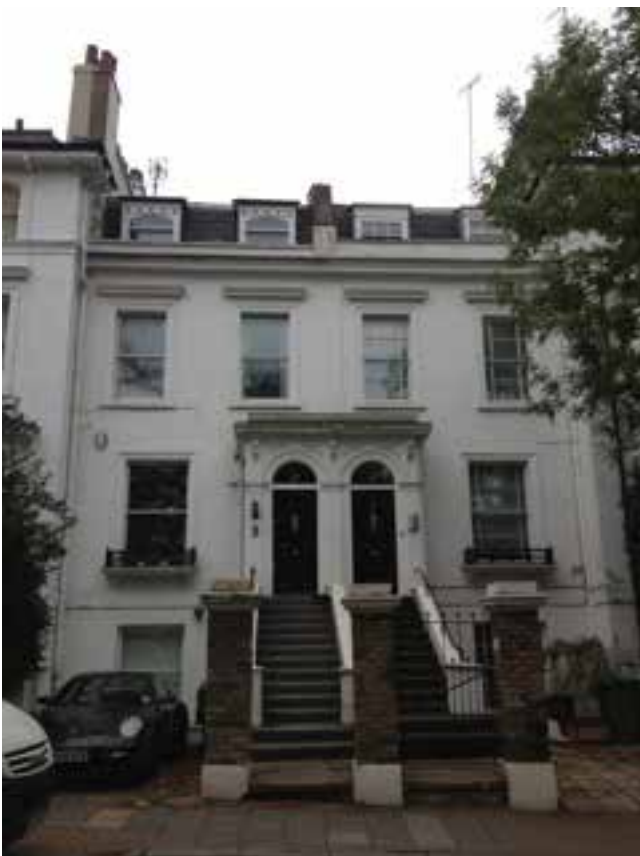
Front view from the street.
