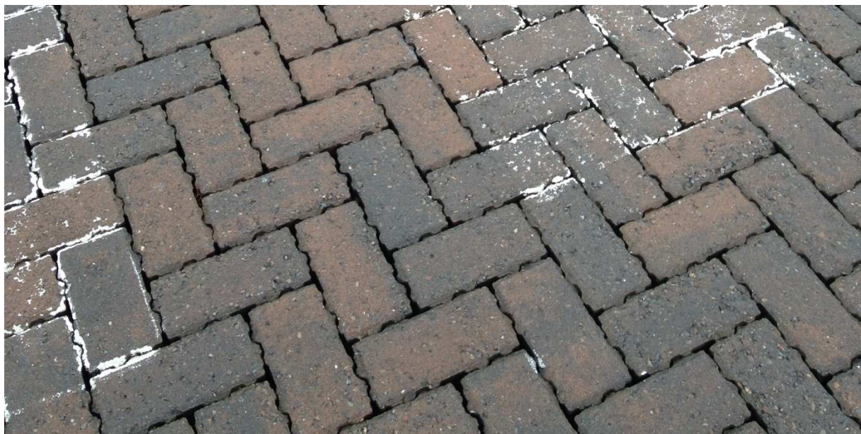
Figure 7 - Typical example of permeable block paving
