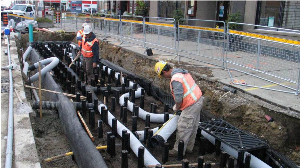
Figure 9 - Photograph of Silva Cell installation
