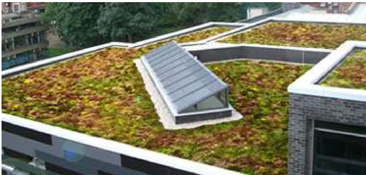
Figure 6 - Typical living roof (reference McLaw Living Roofs)
