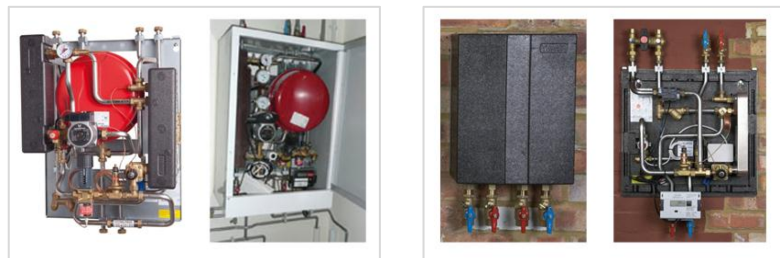
Figure A3.5 – Left: inefficient HIUs. Right: efficient HIUs which will be specified on Agar Grove.
