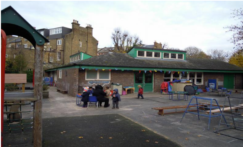
EXISTING NURSERY BUILDING TO BE DEVELOPED INTO NEW EYFS FACILITY
