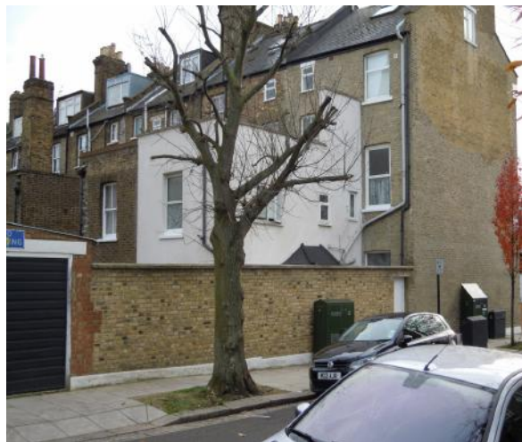
EXISTING HOUSE ON RONA ROAD
