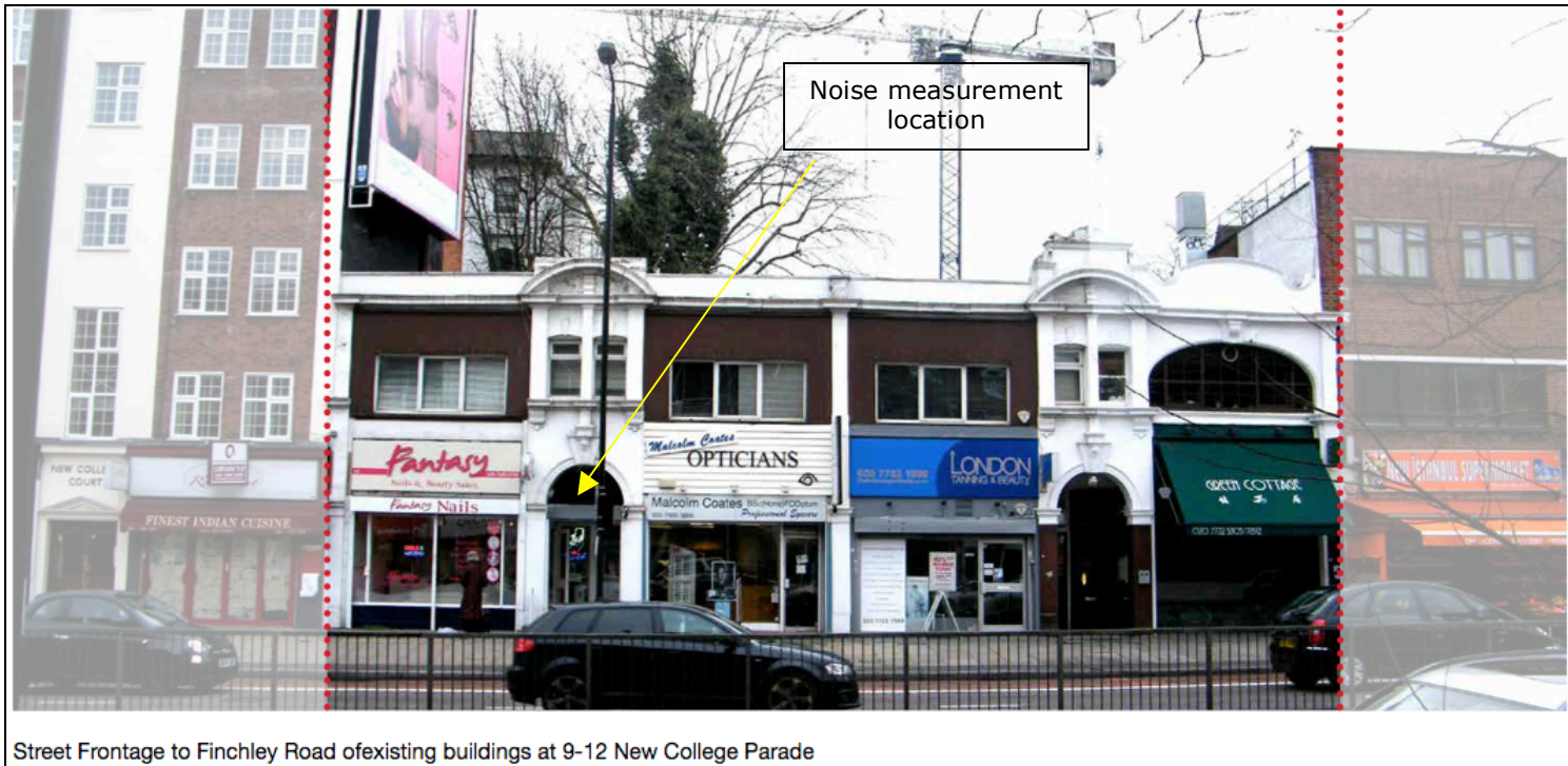
Figure 1 – Existing street frontage
