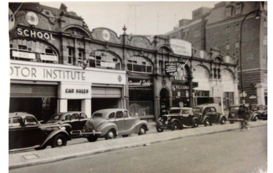
Figure 22: A photograph of the properties at 1-6 New College Parade in the mid 1950s, courtesy of Camden Local Studies Archive. This photograph corresponds with the watercolour shown in figure 23.
