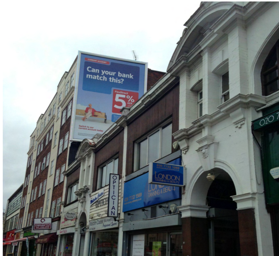
Figure 25: A photograph of the elevation of the properties at 9-12 New College Parade as existing.
