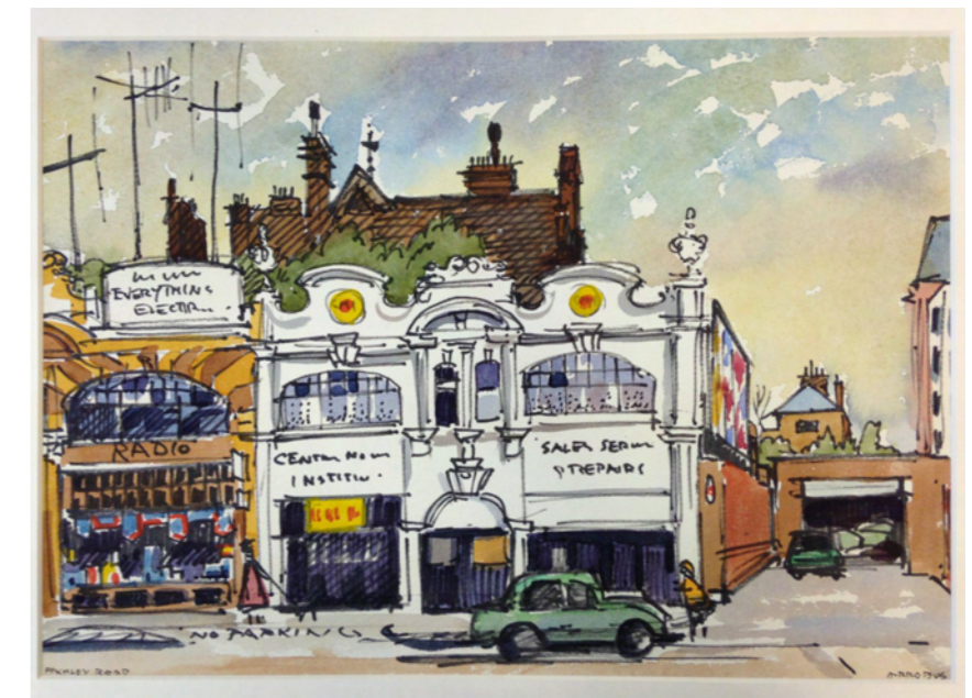
Figure 23: The watercolour produced in the early 1960s which depicts the properties at 1-3 New College Parade. The top of the listed building at 40 College Crescent is visible in the background of this painting. This painting is labelled as being produced c. 1965, although must have been completed just prior to their redevelopment in 1963-4.
