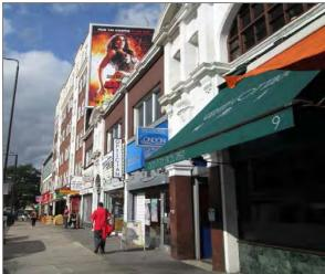
Finchley Road slopes down towards the east and the site is on a number of different levels. The building is cut into the slope of the ground, such that it comprises two storeys with basement at the front and a single storey with double basement at the rear. At the front of the building is a paved pedestrian walkway and at the rear a communal concreted area approximately which is shared with the building to the southeast.
