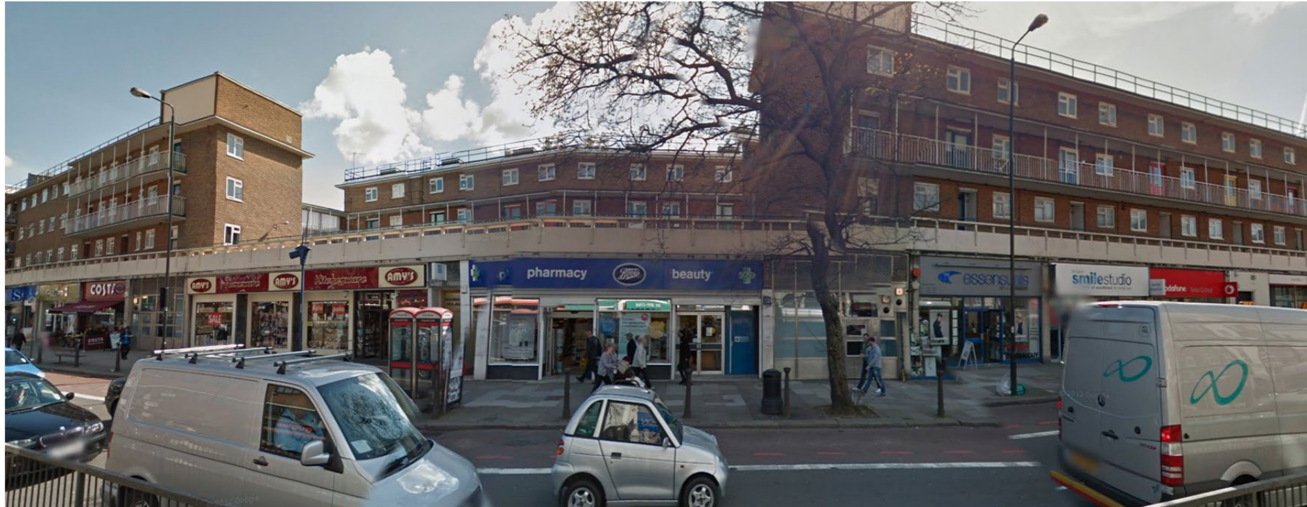
Outlook from front of Existing building
