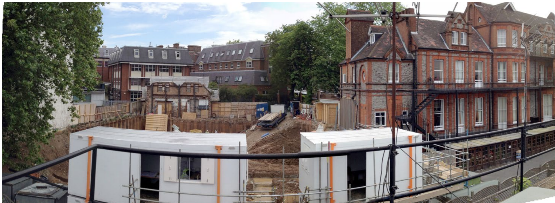
Outlook from Rear of Existing building
