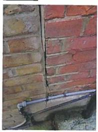
This shows the vertical crack to the left side of the extension at the junction with the main building extending to the ground.
