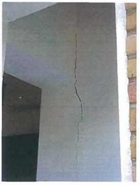
This is a general view of the vertical crack within the single storey extension to the right hand side at the junction with the main building.
