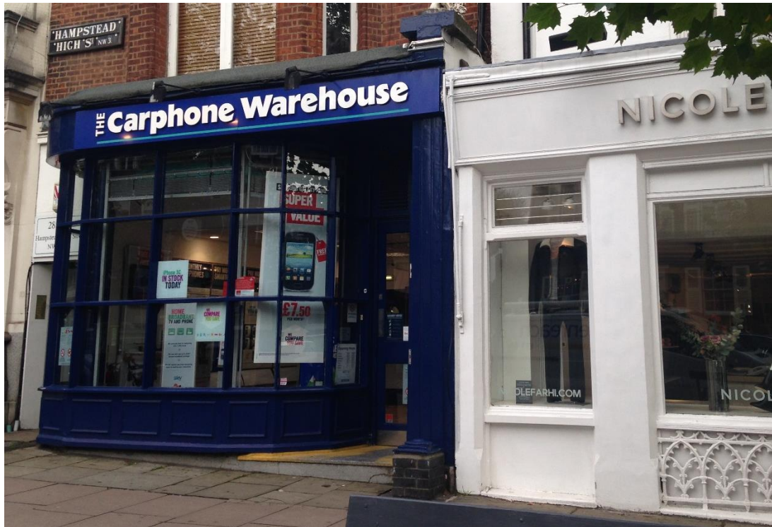
Photo 3: Hampstead Conservation Area – painted timber shopfronts
