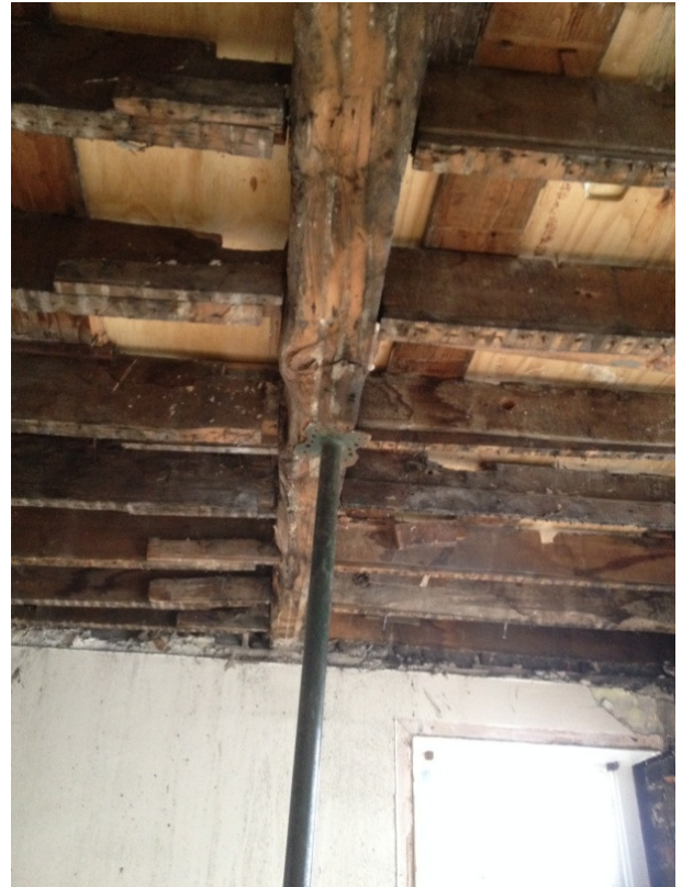
View of existing beam
