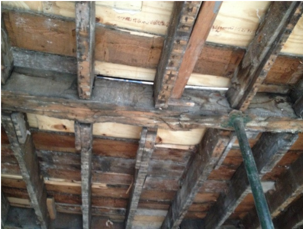
Existing beam propped temporarily
