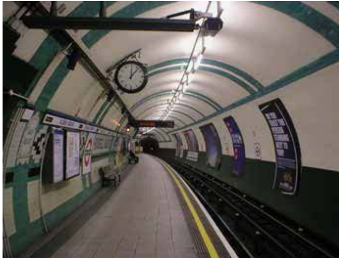
Russell Square Underground Station
