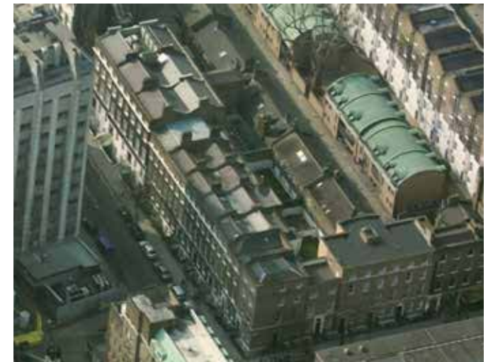
Guilford Street - Aerial view of roof
