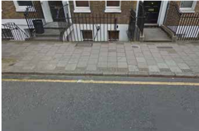
Fig 1.2.20 Pavement along Guilford Street
