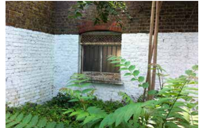
Fig 1.2.14 Wild, unkept rear of site, facing Colonnade properties
