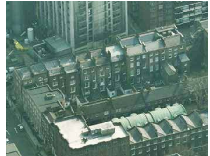
Guilford Street - Aerial view of roof
