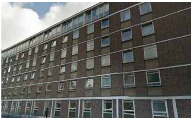
Grenville Street- Looking East
