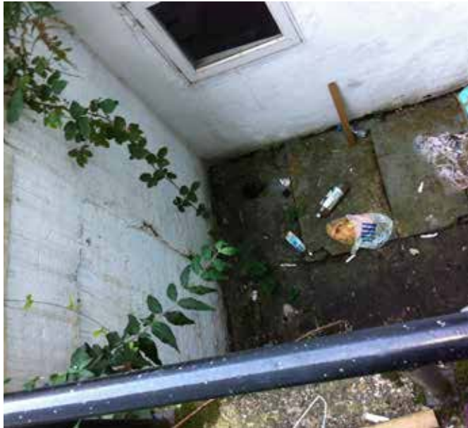
Guilford Street - Rear basement level access
