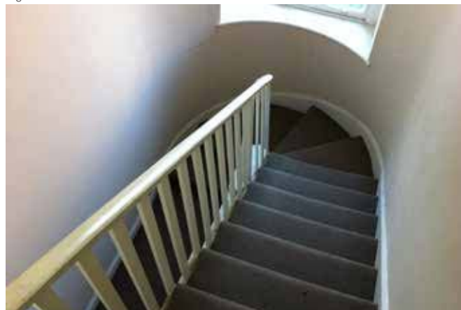
Fig 1.2.13 Guilford Street - Interior staircase
