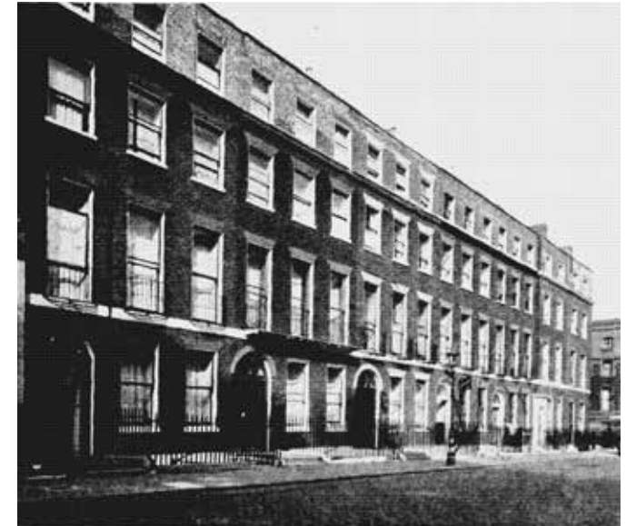
77-82, Guilford Street, Survey of London: volume 24: The parish of St Pancras part 4: King's Cross Neighbourhood (1952), p. 44.
