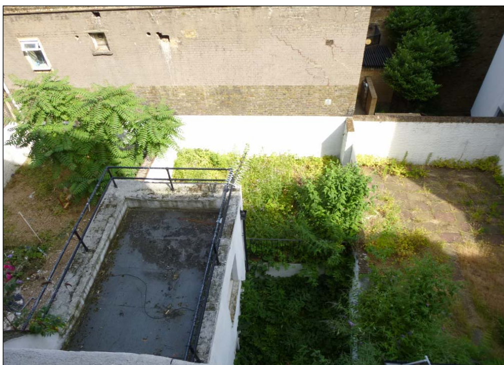
Photograph 6.1: Existing rear extension of Site and its relationships with Colonnade Mews
